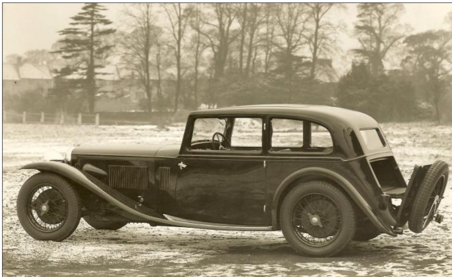
A Vanden Plas saloon photographed when new at the Vanden Plas Works before dispatch, probably a 1933 model. Note the painted 'slave' wheel transit nuts, removed before dispatch. These were popularly known as 'Straight-backed' saloons and Follett sold 28 of them. With the boot lid open, the extending boot floor to carry a trunk may be ascertained.
